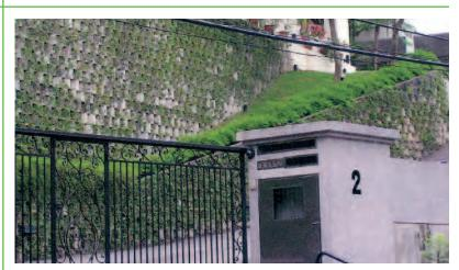
BETOTITAN® walls are fully mono-lithic without intermediate voids adapting well to the difficult terrain and supporting the heaviest loads. The elements are in full contact with each other, having no gaps between them. The soil is held captive within the individual blocks preventing erosion of the soil and weakening of root anchorage.
